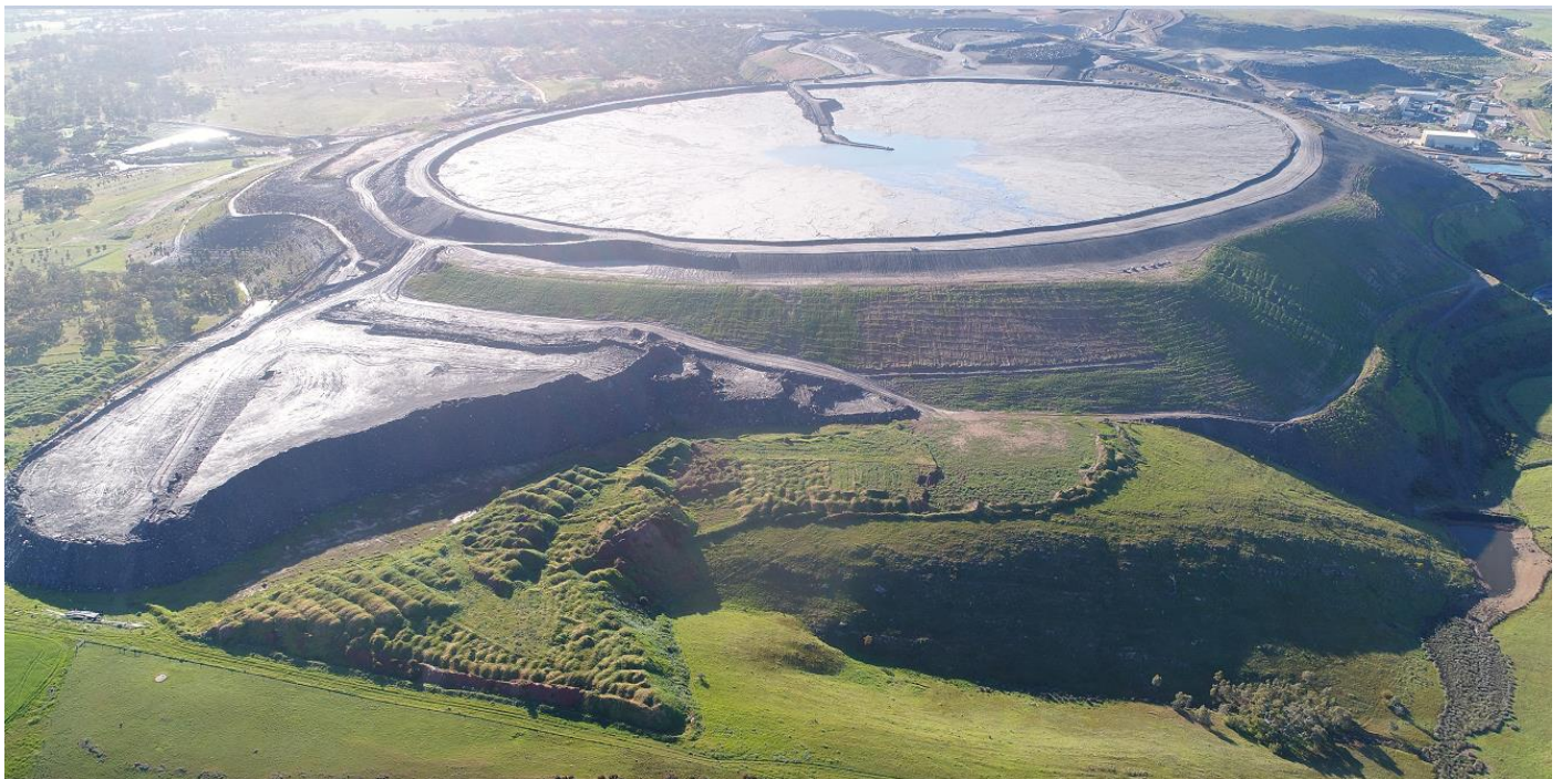
FIGURE 3. REHABILITATION – TSF EMBANKMENTS SEEDED IN MARCH 2019
